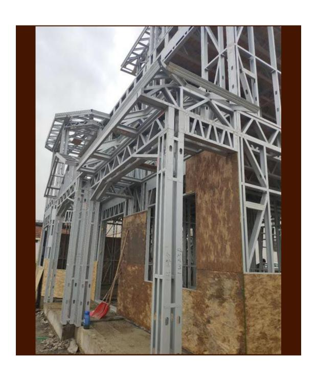
Mass production c profile steel frame made by metal forming machine.
